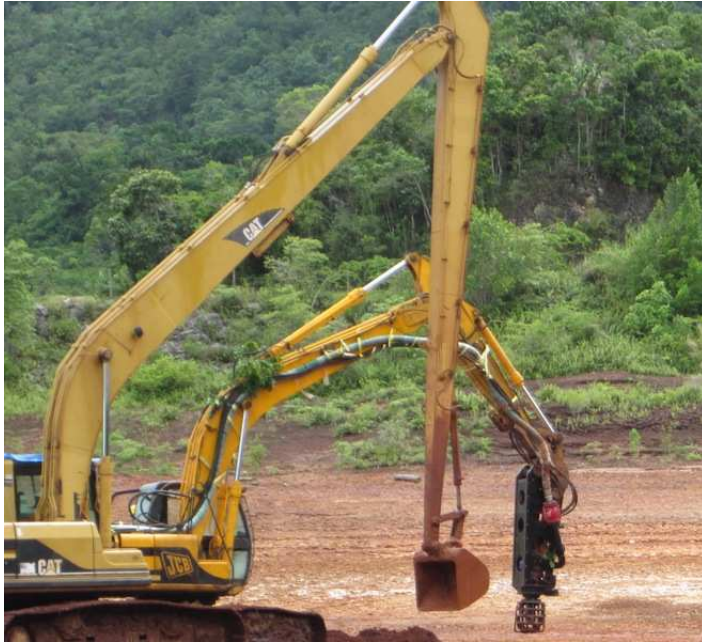
Photo 3.2: CAT 325 Long reach (60ft boom) and JCB220 with Eddy mud pump.
