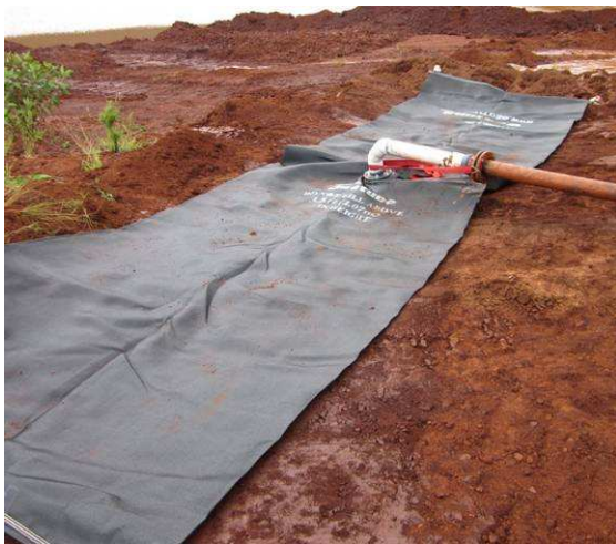
Photo 5.10: Geotube prior to filling
