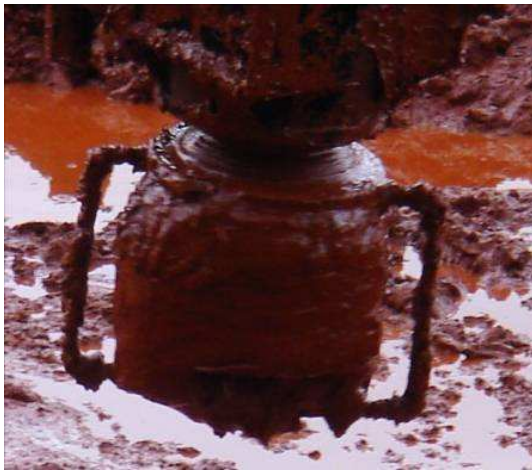
Photo 5.1: Cutter head blinded with mud
