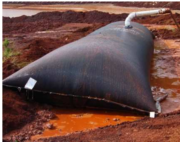
Photo 5.11: Geotube filled taut – note seepage /bleeding
