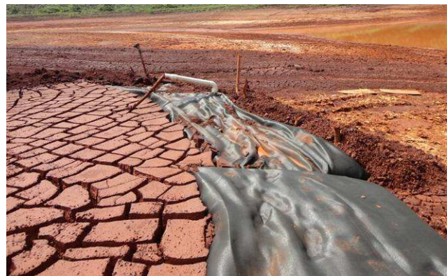
Photo 5.15: Geotube #1 after 6 weeks
