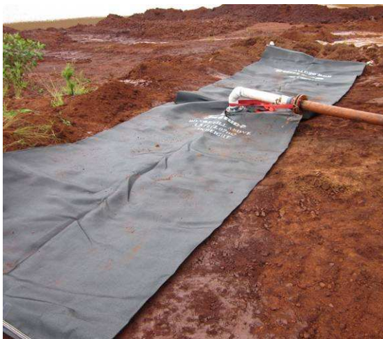
Photo 3.2: Geotube prior to filling
