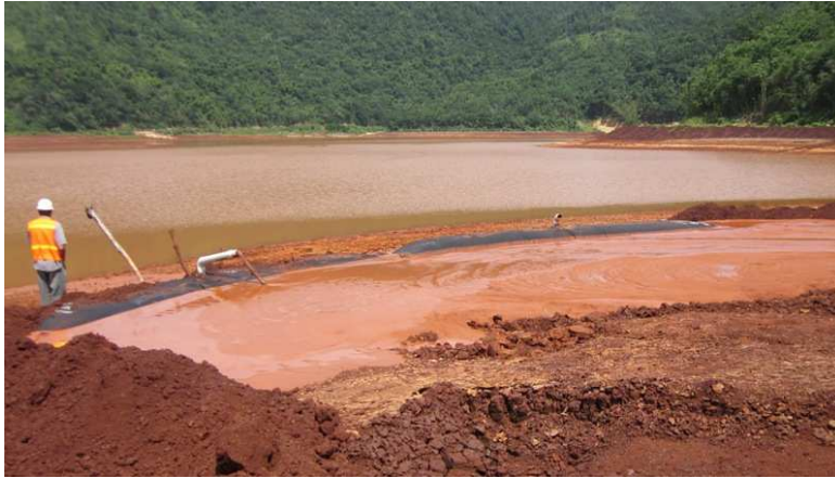
Photo 5.7: Two geo tubes forming the bund of the trial pond
