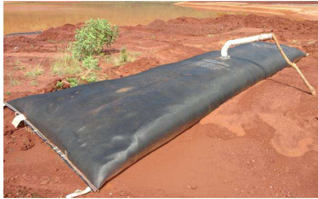
Photo 5.13: Geotube #3 after 6 weeks
