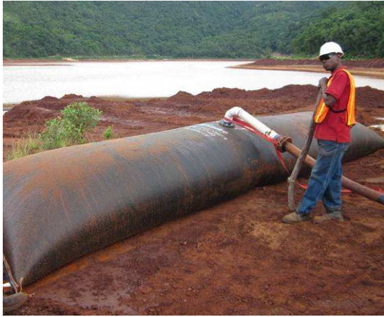
Photo 5.12: Geotube #3 filled to capacity
