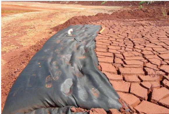
Photo 5.14: Geotube #4 after 6 weeks
