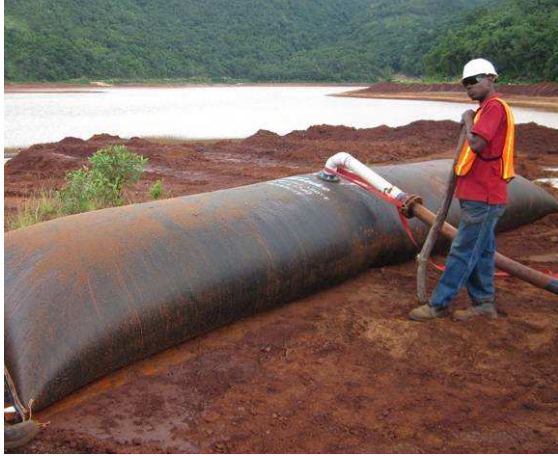
Photo 5.12: Geotube #3 filled to capacity
