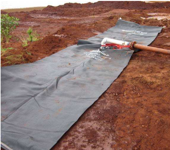
Photo 3.2: Geotube prior to filling
