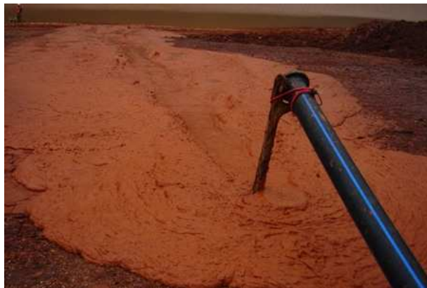
Photo 5.5: Mud discharge point
