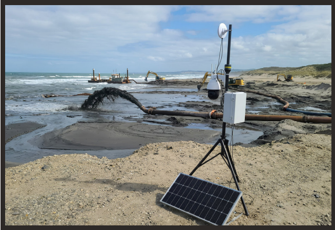
Sediment, slurry, and dewatering outfall observation
