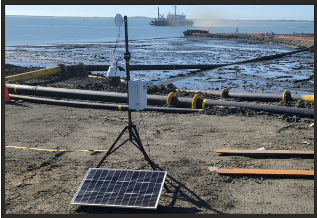
Dredge pipeline discharge monitoring
