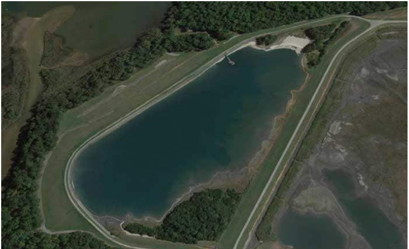
Coal Ash Storage at a Power Plant. Tailings Pond Aerial View.
